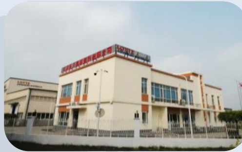
Compounding Plant (Tianjin/Dongguan, China)
